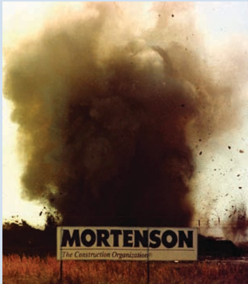
The last U.S. Minuteman II missile silo is imploded in December 1997 in accordance with START.
